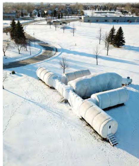
The Inflatible Lunar/Mars Analog Habitat (ILMAH) has five modules: the living quarters module, a botany/greenhouse module, geology module, exercise module, and an extravehicular activity (EVA) module. Docked to the ILMAH via a tunnel is the Pressurized Electric Rover (PER), which students used to conduct EVAs outside of the habitat.
