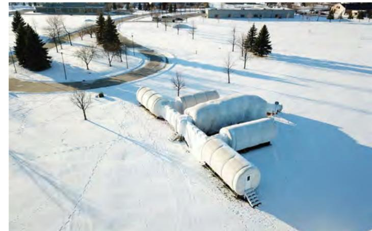
The Inflatable Lunar/Mars Analog Habitat (ILMAH) has five modules: the living quarters module, a botany/greenhouse module, geology module, exercise module, and an extravehicular activity (EVA) module. Docked to the ILMAH via a tunnel is the Pressurized Electric Rover (PER), which students used to conduct EVAs outside of the habitat.
